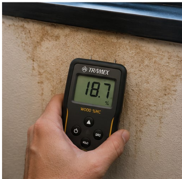
IEQ-01C · MEASUREMENT LOCATION Adjacent wall finish
