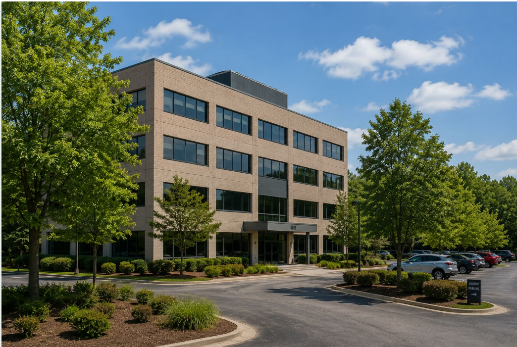
EXAMPLE PROPERTY · Commercial Office Building
